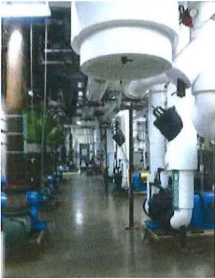
Chilled Water System
