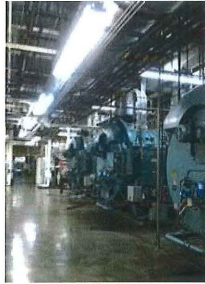
Steam Boiler System
