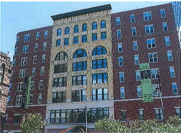
Main & Temple Apartments
