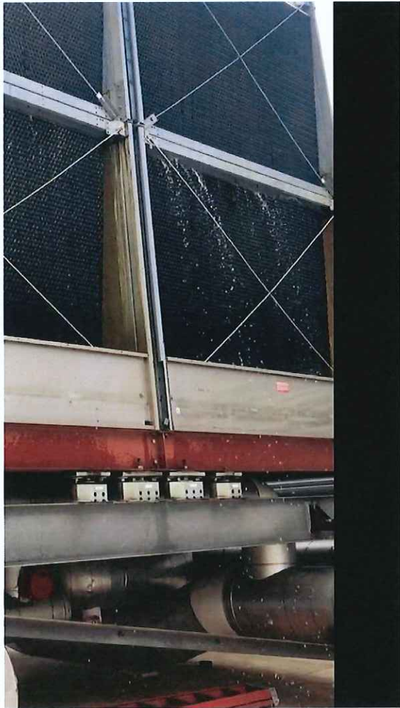
Water leaking out of bowing cooling tower wall media
