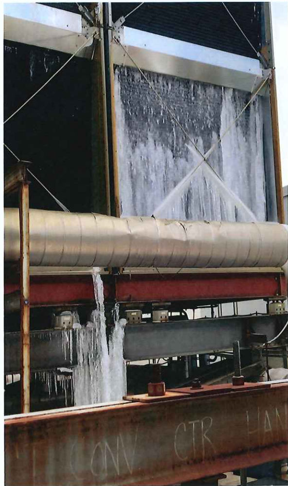
Frozen water seized up cooling tower wall media
