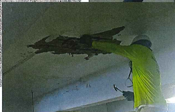
Full Depth Repair in Progress
