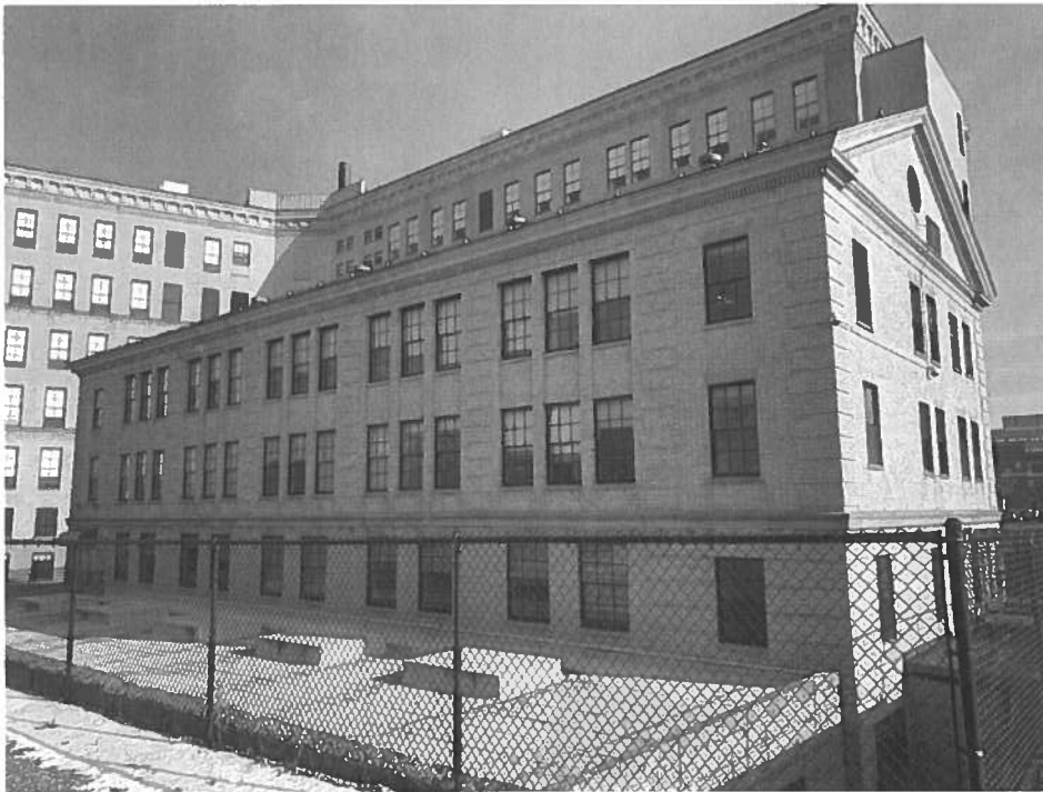
This annex building connected to the main building at 55 Elm will also be converted to apartments. It's ground level may become a destination such as distillery, brewery, bakery or coffee roasterie. (Kenneth R. Gosselin / The Hartford Courant)
