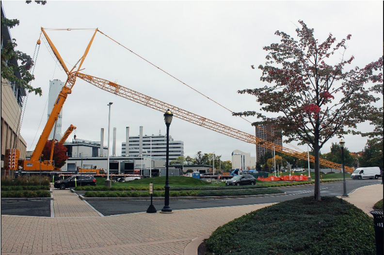
Crane positioned to replace Chilled Water-Cooling Towers
