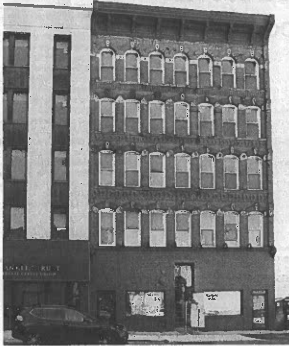
Jose Ramirez converted the upper floors of 289 Asylum St. (shown above) in downtown Hartford to condos that he is currently renting.
