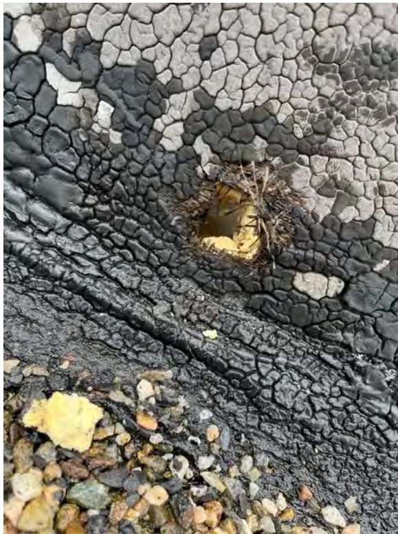
Building 2,3,4,5 – Representative ACM four ply asphaltic roof membrane
