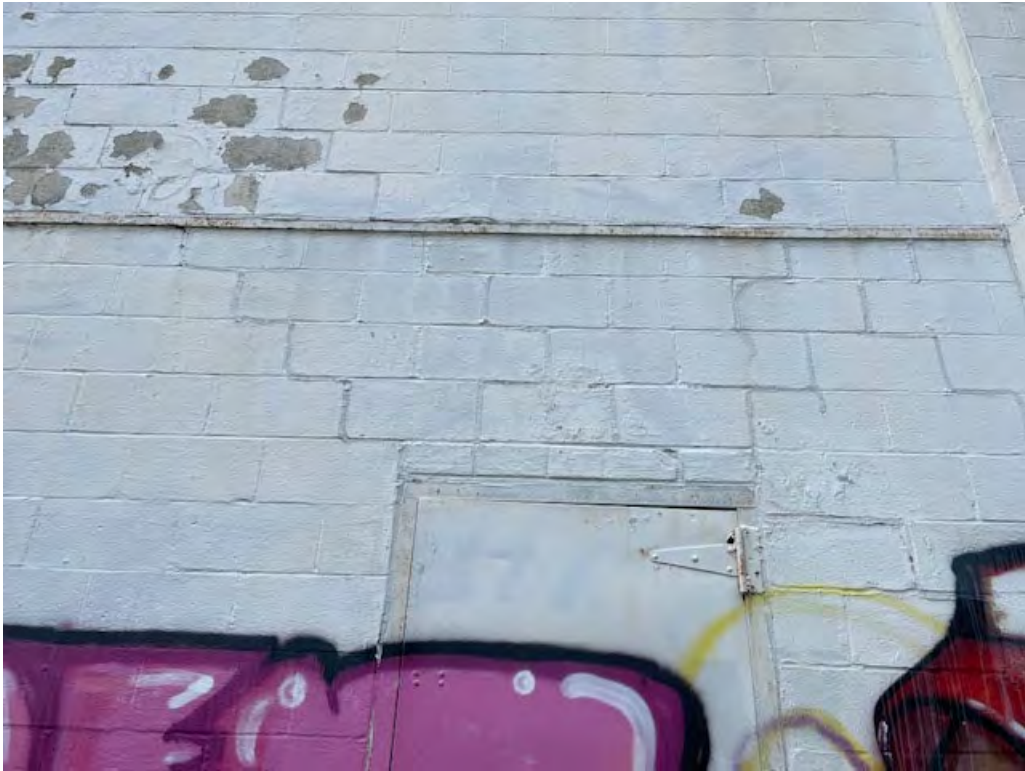
Building 2 - ACM horizontal joint caulks - grey original and white repair caulk
