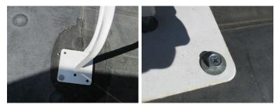
Steel flanges for a rooftop mechanical unit support frame are screwfastened directly through the roof membrane, with no means in place to make the fastener penetrations through the roof membrane watertight.
