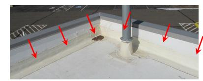
When the overlay roof covering systems were installed (in 2020), the new EPDM roof membrane was turned up onto the face of perimeter parapets. and flashed with a strip of self-adhering flashing membrane (see arrows). Edges of the flashing membrane are caulked with elastomeric sealant.
