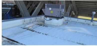
There are numerous rows of metal pipe stanchions, for anchorage of rooftop safety railings on the roofs (Buildings 1-9), that have no safety railings attached (photos above/below)
