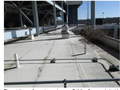
The existing roof covering systems on Building 8 appear to be identical to those on Buildings 2, 4-7, and 9, in type and construction, with the exception of one small addition (Roof Area 8-D), that utilizes an adhered EPDM single-ply membrane system.
