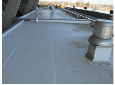
Overview of the roof on a typical Concourse-Level building (Building 4 shown here). The TPO single-ply membrane roof covering system on this building is from original construction of the facility.
