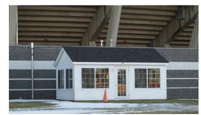
The Catering Building visually appears to be a factory-fabricated and delivered building. The building rests on grade, and it utilizes wood framing, vinyl exterior siding, and plywood or OSB roof deck sheathing. The roof covering system utilizes laminated asphalt/fiberglass shingles that are nailed (presumably through a felt underlayment), to the roof deck.
