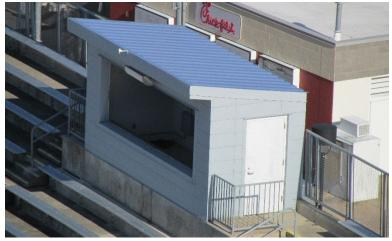
The Video Booth is located at the top of the upper bowl. off the east end zone. The "shed" building appears to be constructed with light-gauge steel stud framing, and utilizes a pre-manufactured pre-finished metal panel roof covering system that is mechanically fastened to the roof framing (similar to that on the Scoreboard Roof).
