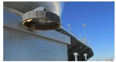
The kitchen grease container, which is normally attached to the screw-top flange, appears to be broken off or missing from this exhaust fan unit (Building 3), thus potentially allowing food grease to drip onto the roof surface, causing damage.
