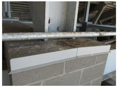
The acidity of bird droppings causes damage to paint/finishes on sheet metal flashings, as well as conduits and steel structural members. Once the paint/coatings on metals/steel are eroded through, bird feces typically will cause corrosion of the underlying metal/steel.
