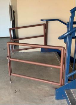
Figure 6: Gates at stair discharge level
