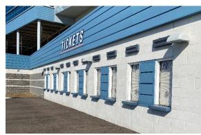
Determine current ticket office requirements; windows are rusted, rotting and sealant and signage is deficient and at end of life
