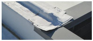
TPO membrane, at ends of an expansion joint cover, is loose/detached/ non-watertight.
