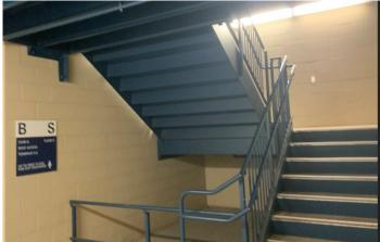
Figure 4: Bottom landing of stair without sprinkler coverage
