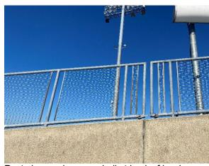
Rust observed on guardrail at back of bowl
