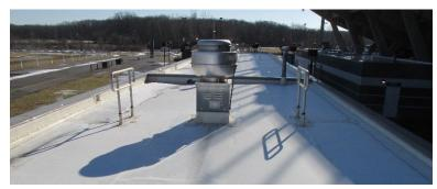
Sections of safety railings are installed adjacent to some rooftop mechanical units, as fall protection (photos above/below); the railings are anchored to metal pipe stanchions that are flashed with EPDM membrane
