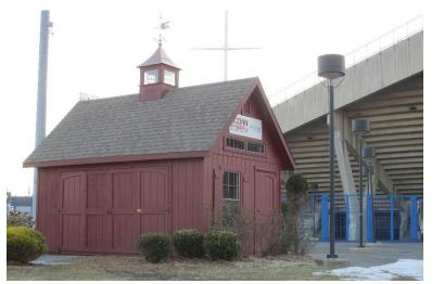
The Radio Broadcasting Building (also referred to as "The Dog House") is a wood-framed building with T1-11 exterior siding and (presumably) plywood roof deck sheathing. The roof covering system utilizes laminated ("architectural") asphalt/fiberglass shingles that are nailed (presumably through a felt underlayment), to the roof deck. A metal-clad cupola is constructed at the center of the roof ridge.
