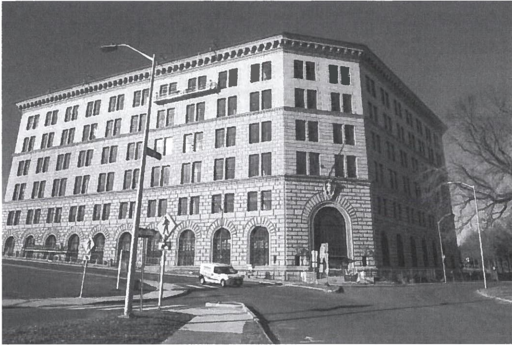
The former state offices at 55 Elm St, in downtown Hartford have been converted to apartments. (Aaron Flaum/Hartford Courant)
