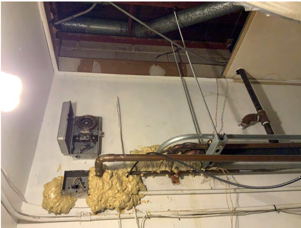
ACM tape & joint compound (throughout)
