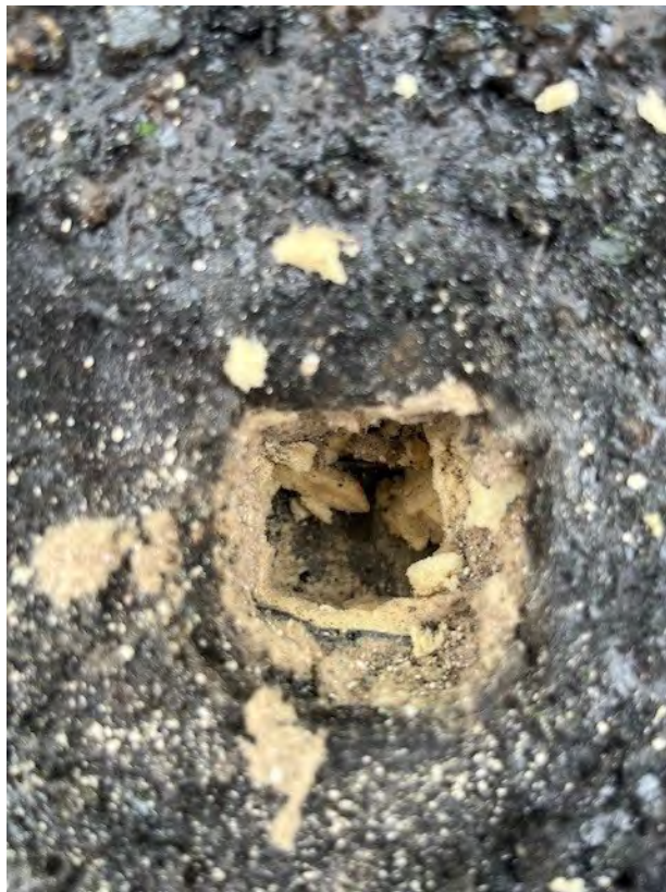
ACM Black 4-ply roof field/ flashing throughout both building roofs
